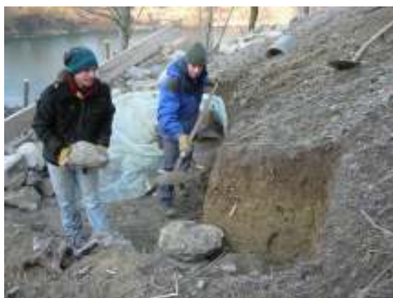
Steinlinsenbau in Ossingen
